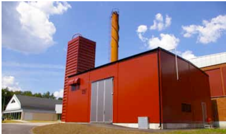
Pellet DHP in Gislaved 17.000.000 Btu for a school, sport arena and community district heating.
