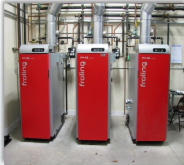
Cord Wood Boilers
