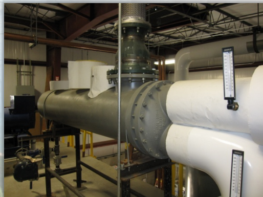
Steam to hot water heat exchanger
