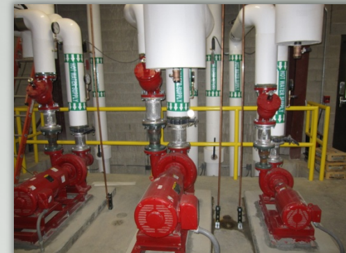
HX and Distribution Pumps to three facilities
