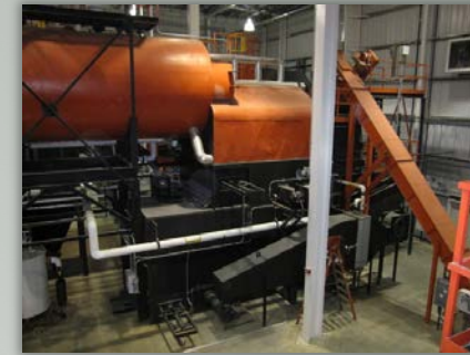
Wood Chip Boilers
