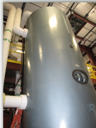
6,000 gallons thermal storage
