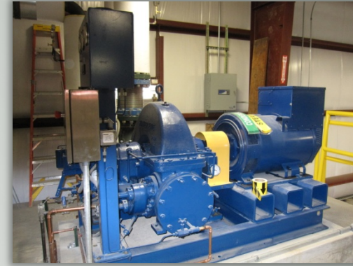
200 kW turbine/generator
