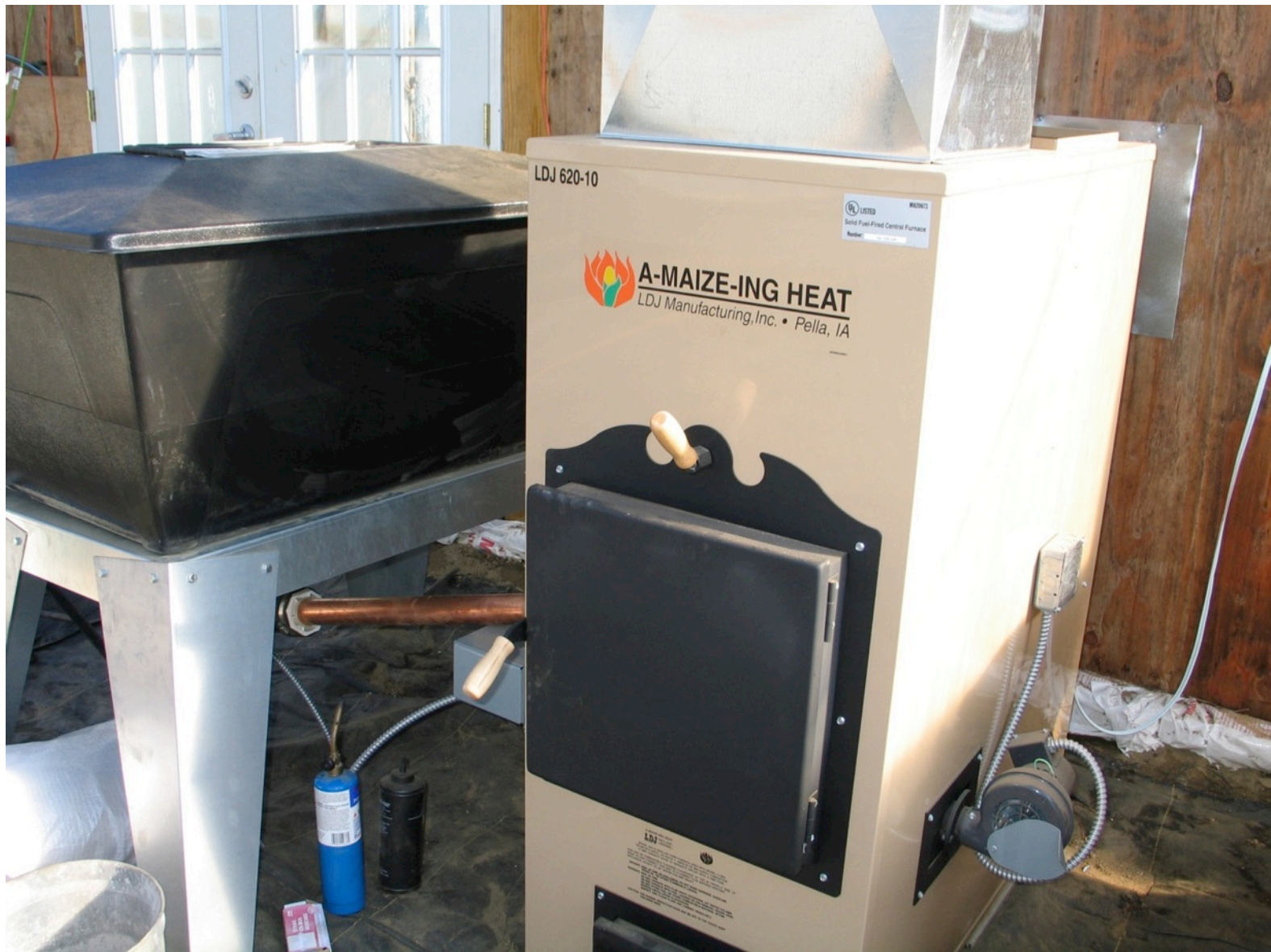
Pellet furnace/boiler ~165,000 Btu
