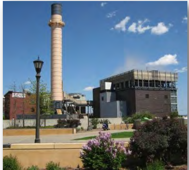
Biomass Fired CHP in Downtown Saint Paul
