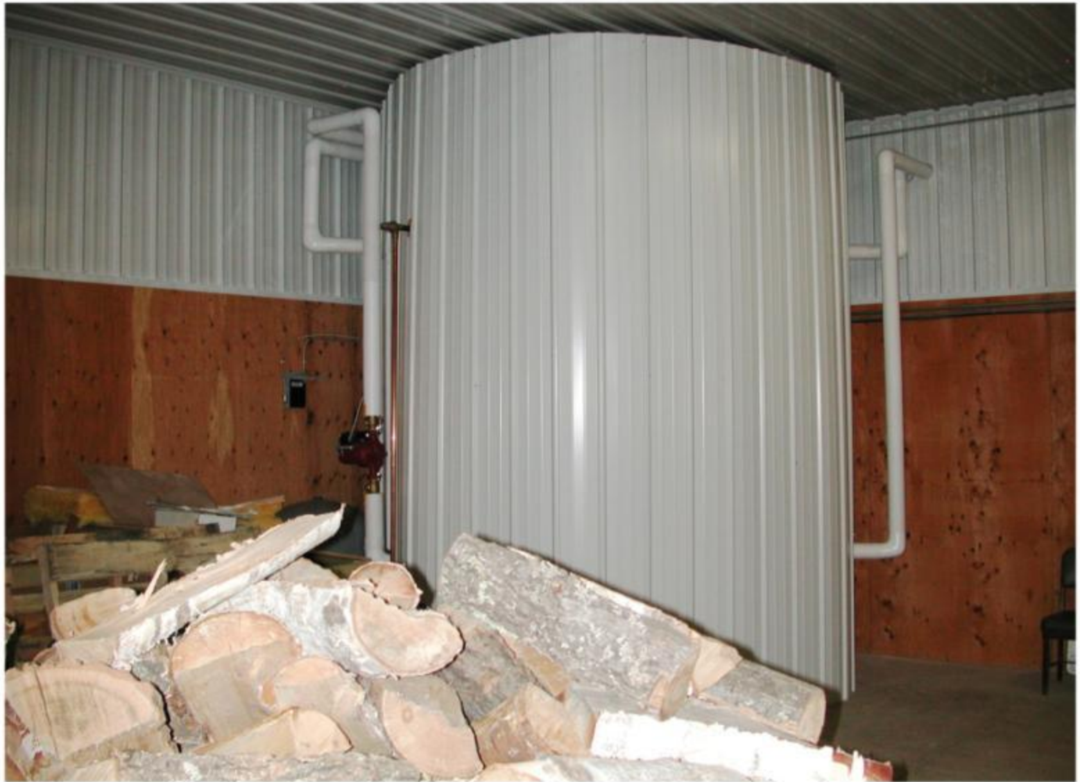
Wood Gun 4000 gallon storage tank
