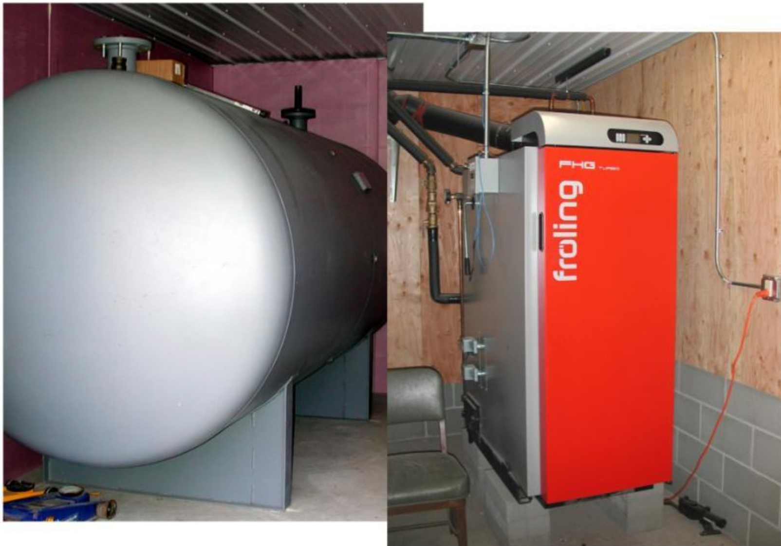
Frohling with 1600 gallon storage tank
