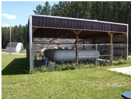
Propane storage currently used by Sawyer Community Center, Sawyer
