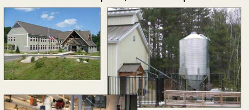
40 Ton Pellet Silo w/ Automatic Auger Feed to a 4 Ton Day Bin/Hopper inside
