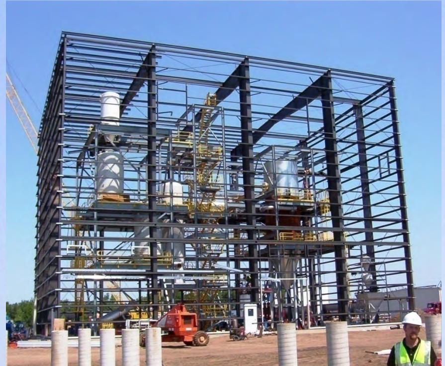
Construction at CVEC August, 2007
